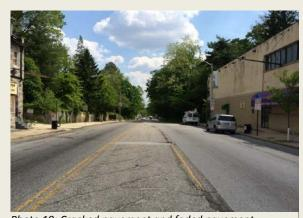
Photo 19: Cracked pavement and faded pavement markings
