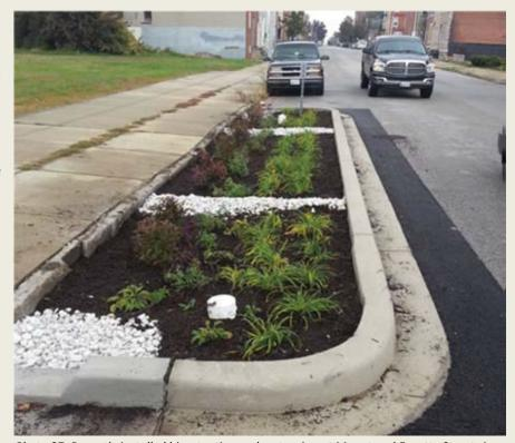
Photo 27: Recently installed bioretention curb extension at Mount and Fayette Streets in West Baltimore
