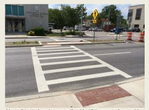
Photo 31: Updated crosswalk with ADA ramps, detectable warning surface and pedestrian refuge
